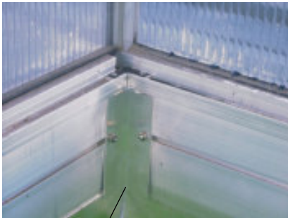
Angle Brackets on the Foundation Frame
